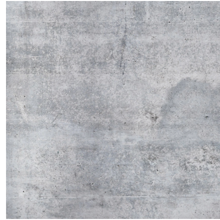
EXPOSED CONCRETE (CONCRETE CURBS)
