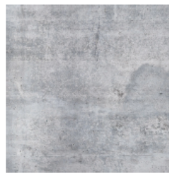
EXPOSED CONCRETE (CONCRETE CURBS)
